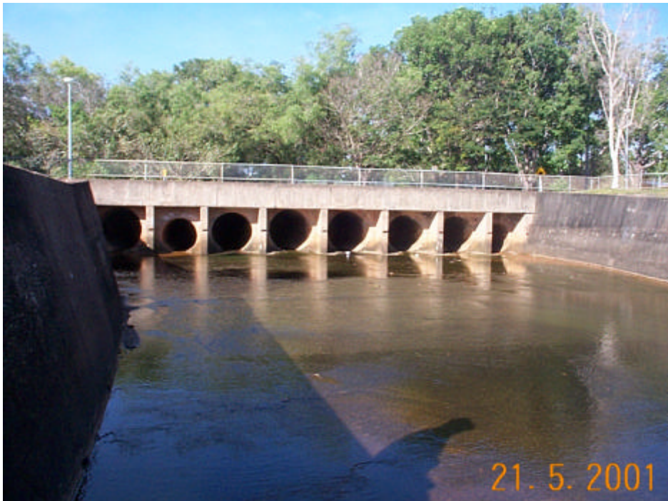
■ Figure 3.1: Upstream end of concrete lined drain showing culverts. Note low dry season flow.
