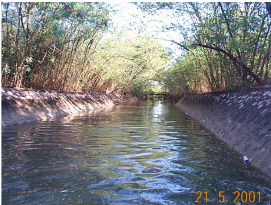
■ Figure 3.4: View of lower end of formed drain on rising tide, with lower footbridge in distance. Note thickets of coffee bush on both banks.
