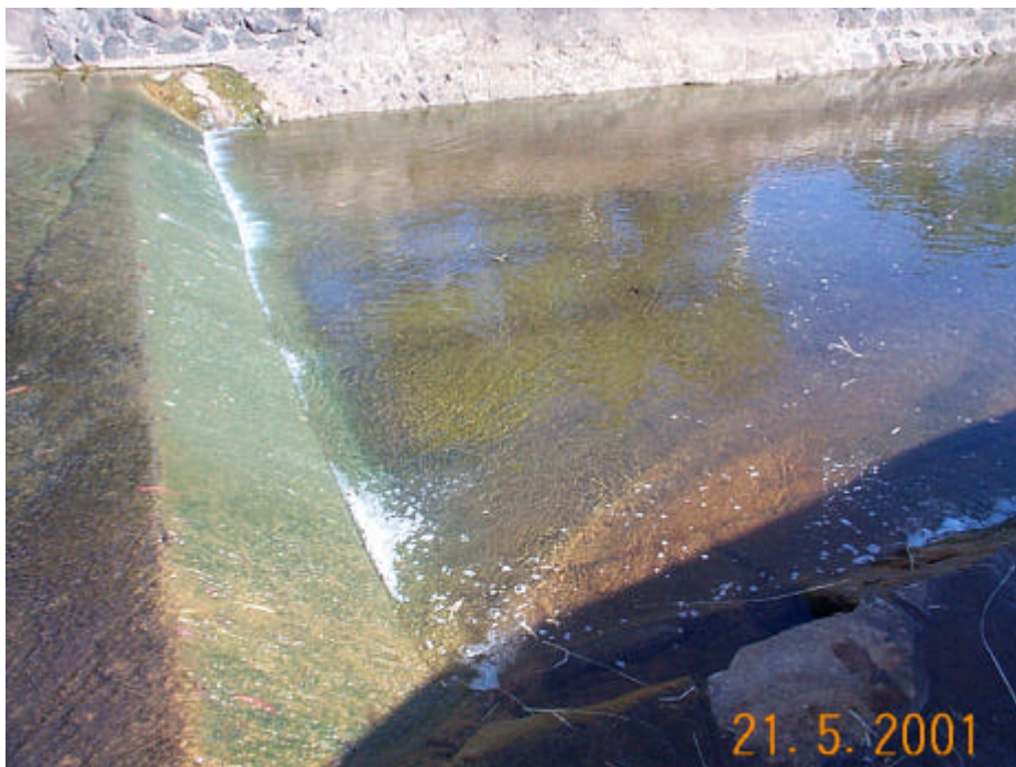
■ Figure 3.2: Step in drain downstream of culverts. Note presence of film of algae on substrate above and below step.
