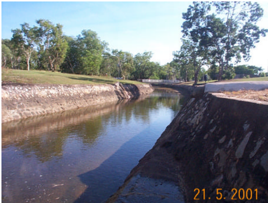
■ Figure 3.3: View looking downstream toward footbridge at low tide, dry season.
