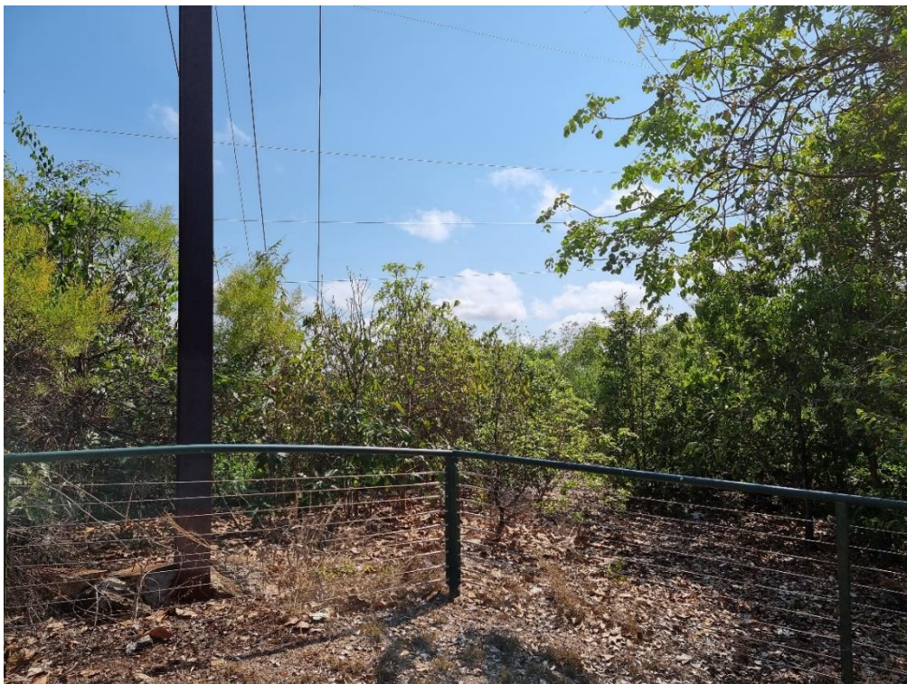
Fig. B4 Fence corner post is “Point Y” at the east end of the southern boundary to Lot 7651
