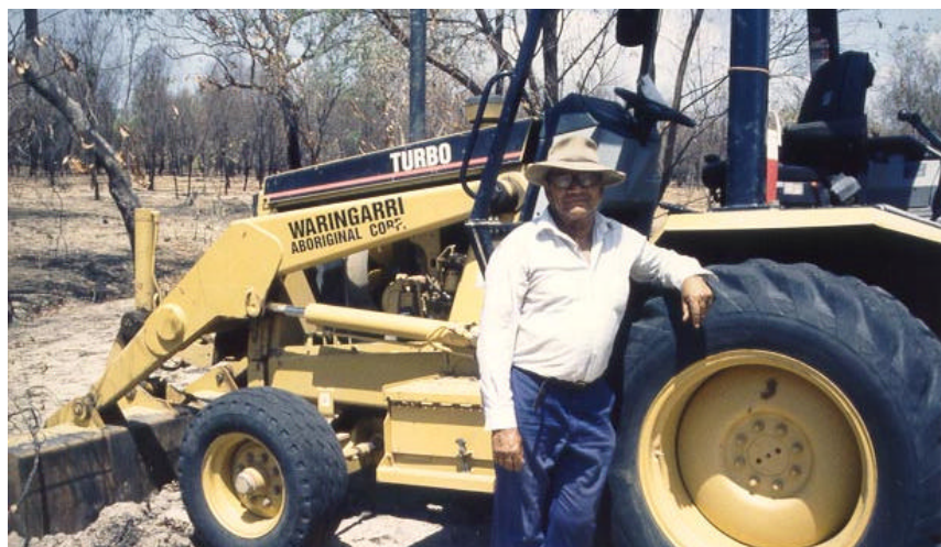
Figure 12.6 Jack Trust, Waringarri machine operator during the 1998 geotechnical investigation work
