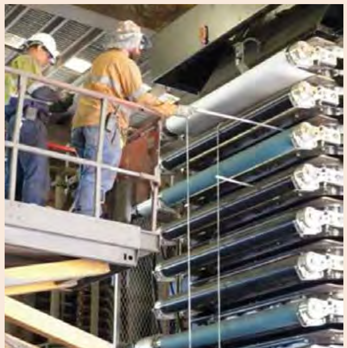
Filter cloth is installed on the new Filter 1 by Jim Rego from Outotec and Scott Walter from Blue Sea Cranes.
