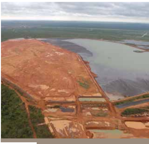
Cell One is undergoing rehabilitation work, which has included installation of a 500mm clay cap.
