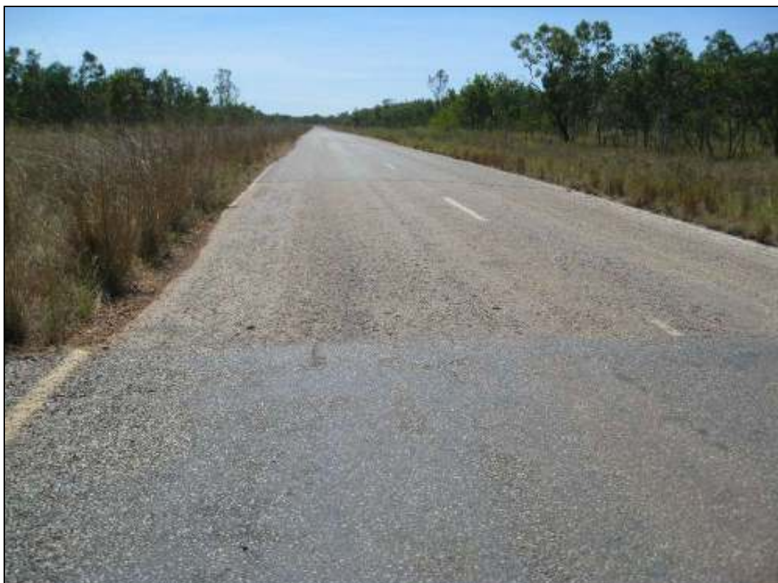
Figure 4 Example of uneven surface and incorrect camber
