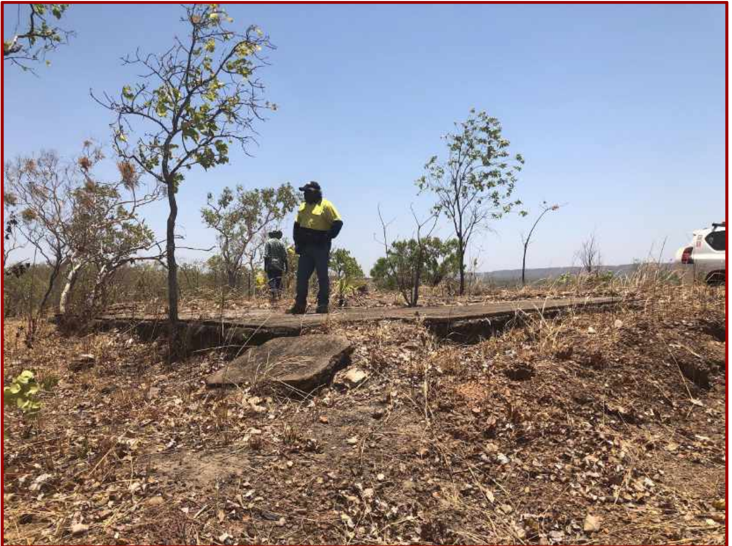
Figure 61: One of the concrete slabs on the ridgeline
