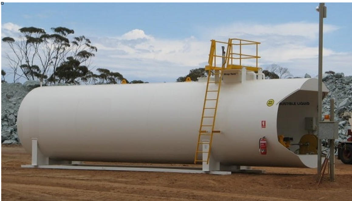
Plate 4.7 – Typical Self Bunded Fuel Storage Tank
