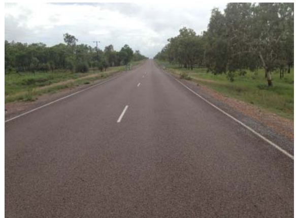
Plate 4 Arnhem Hwy - two-way, single lane sealed roadway section, 122km from Jabiru
