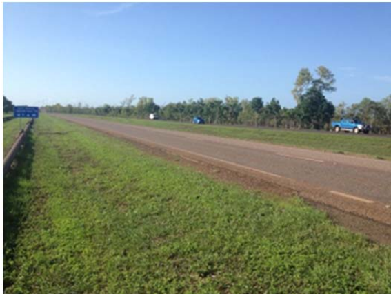
Plate 1 Stuart Hwy - two-way, four lane sealed roadway separated by vegetated median, located 31km from the Berrimah Road intersection
