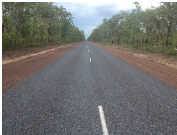
Plate 6 Kakadu Hwy - unsealed clear-zone 30km from Jabiru
