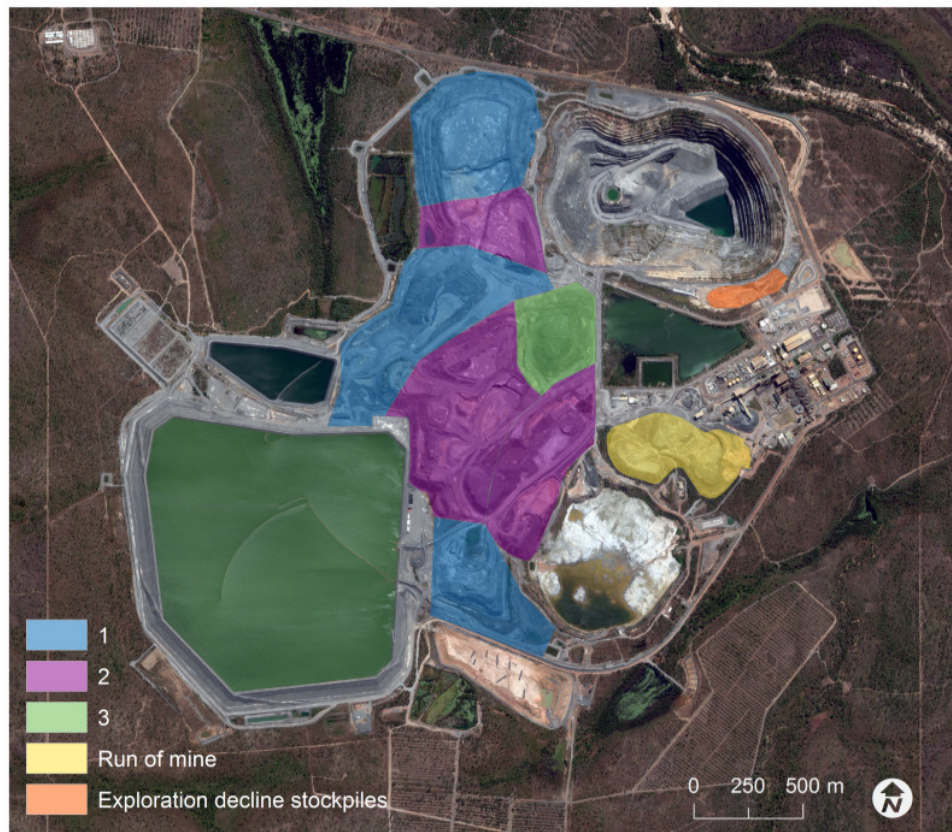
Figure 2-26: Ranger stockpile locations
