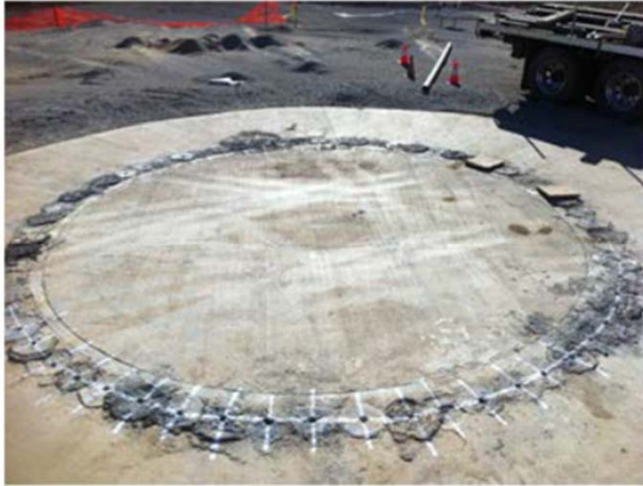
Figure 3-22: Ventilation shaft slab showing completed pile driving
