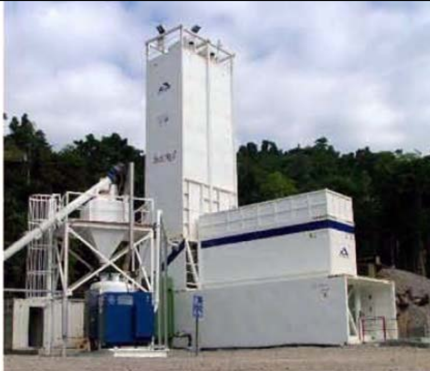
Figure 15: Typical surface backfill plant
