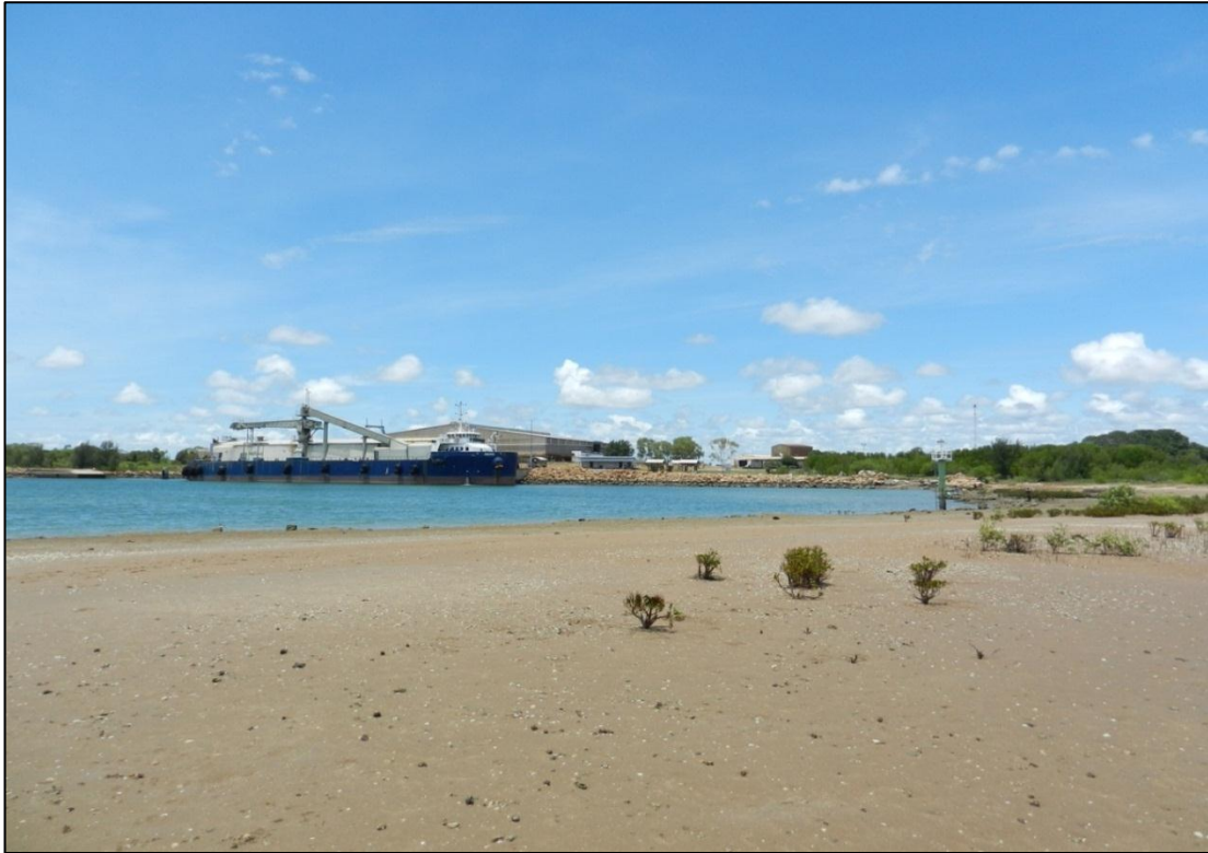
Figure 5-3 Facing South-East Toward Proposed Barge Landing Facility and Existing Xstrata Facility
