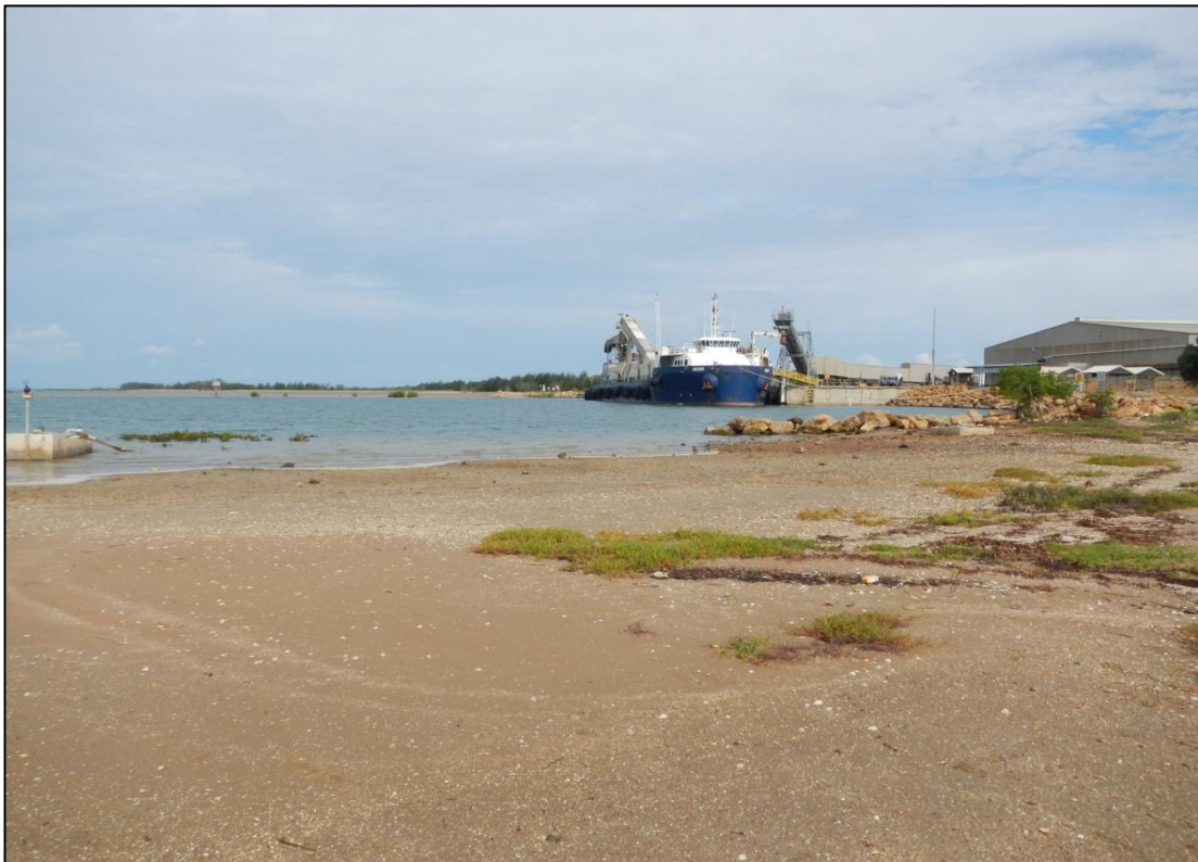
Figure 5-4 Facing South Toward Proposed Barge Landing Facility and Existing Xstrata Facility
