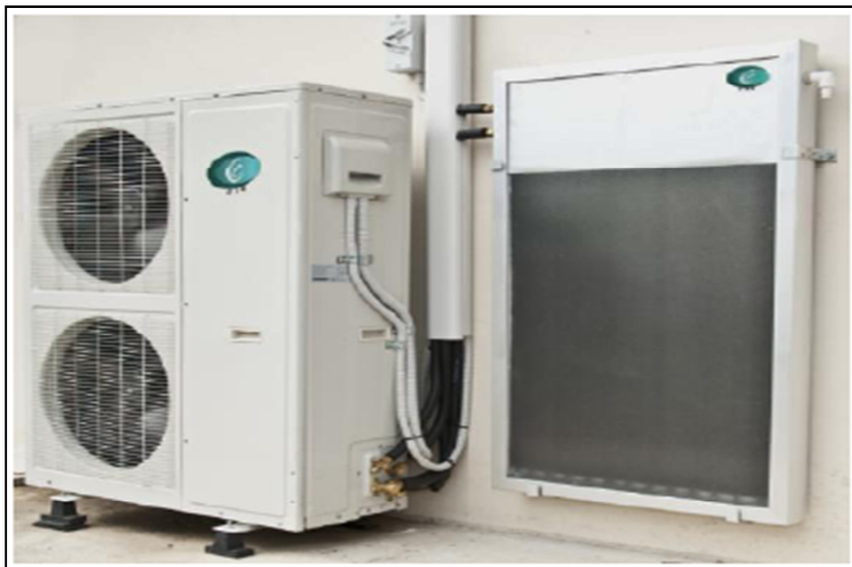
Figure 7-25 – Solar Thermal HVAC
