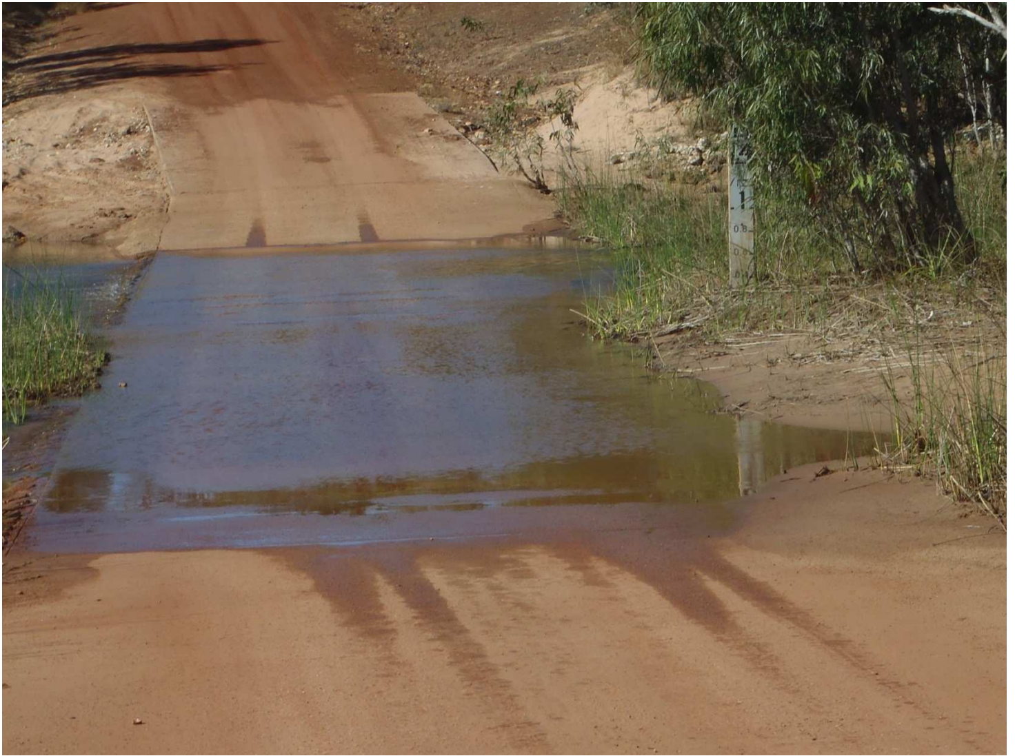
Towns River crossing at Savannah Way.
