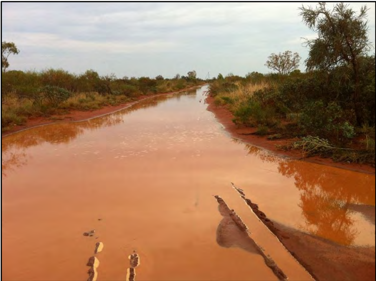
Figure 6: Access Road to the Mine Camp (flooded following a 62mm rain event).
