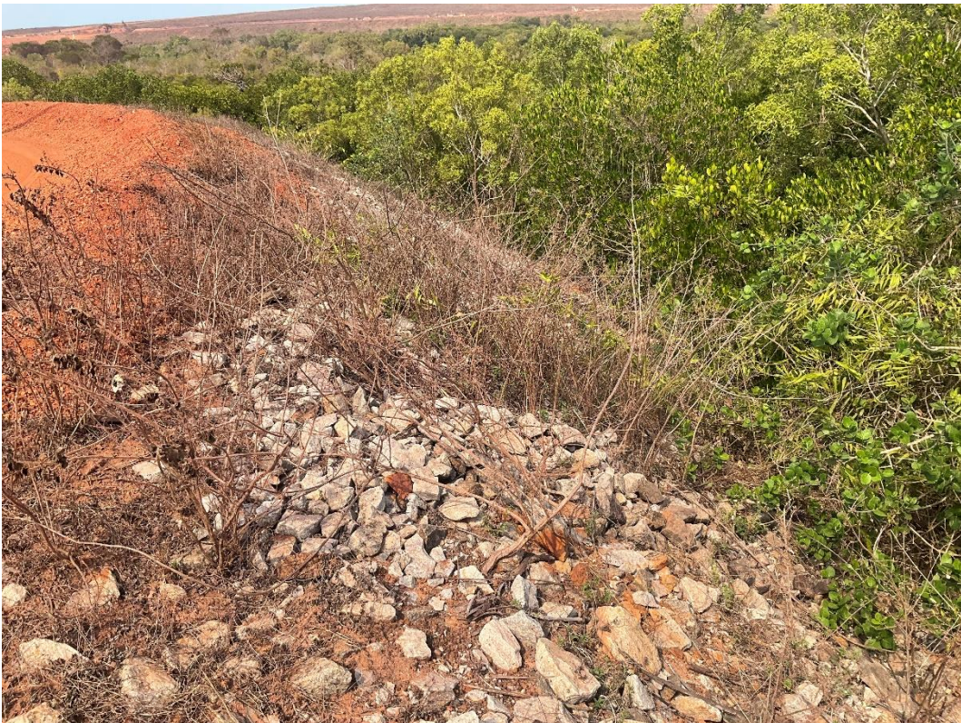
Figure 8: Exotic rubble on slopes of Pond 2.
