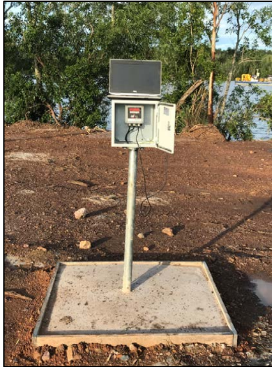
Figure 5-2 – completed VWP and data logger installation at drillhole 18DH02
