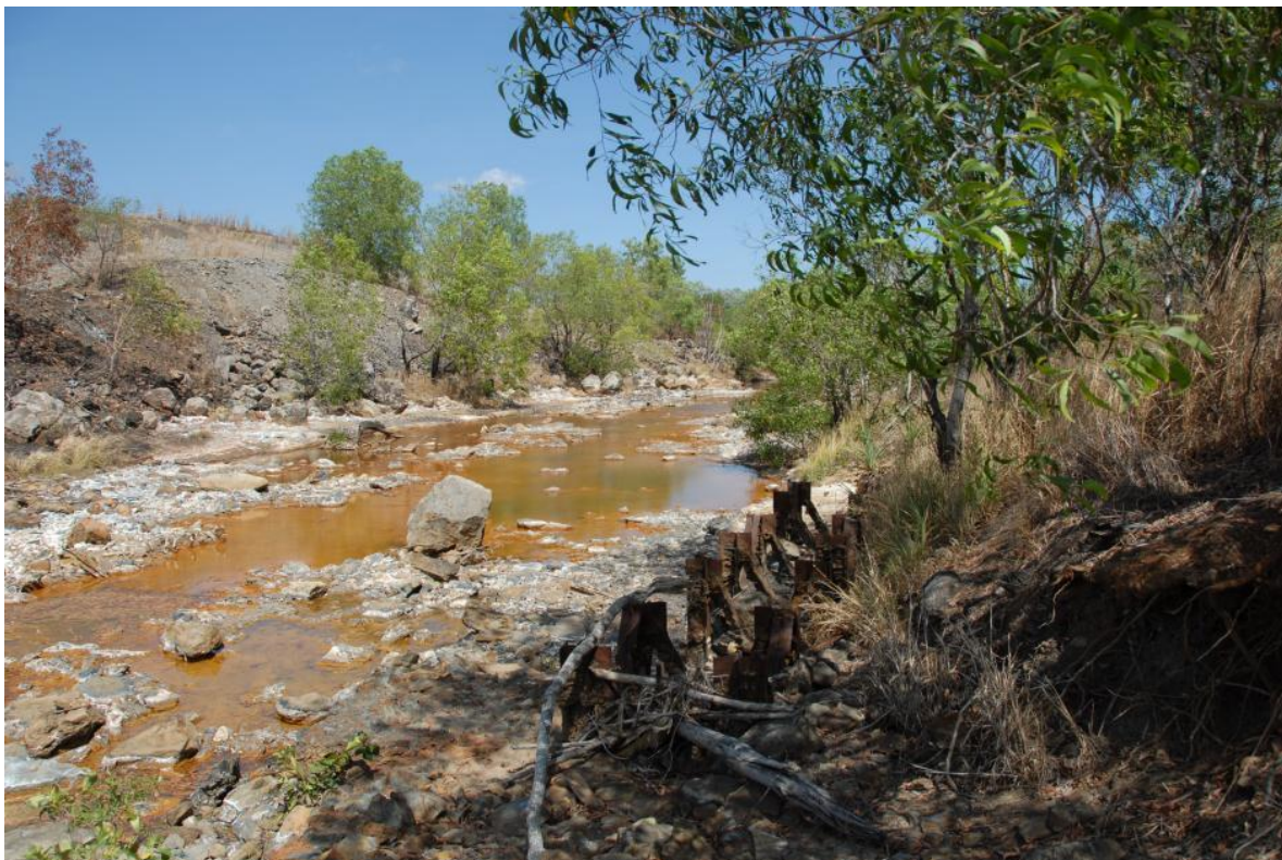
Plate 2 Salt efflorescence and seepage in the diversion channel at the toe of Intermediate waste rock dump, Rum Jungle (NT DME)
