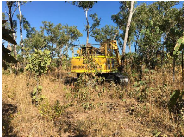
STP-03 Looking South
