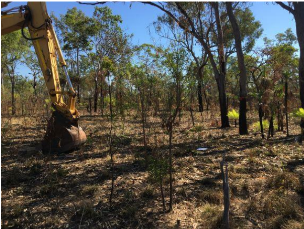
STP-06 Looking West
