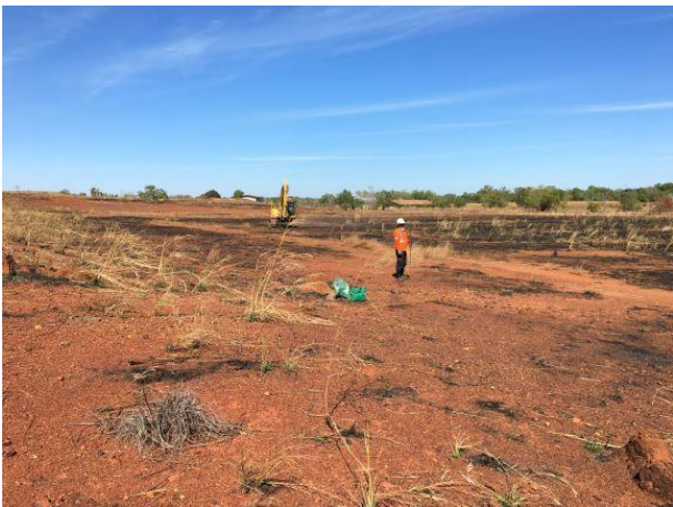
At WRTP-03 looking south across Old Tailings dam with remanent structures in background
