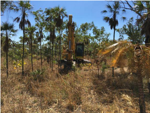
STP-01 Looking North
