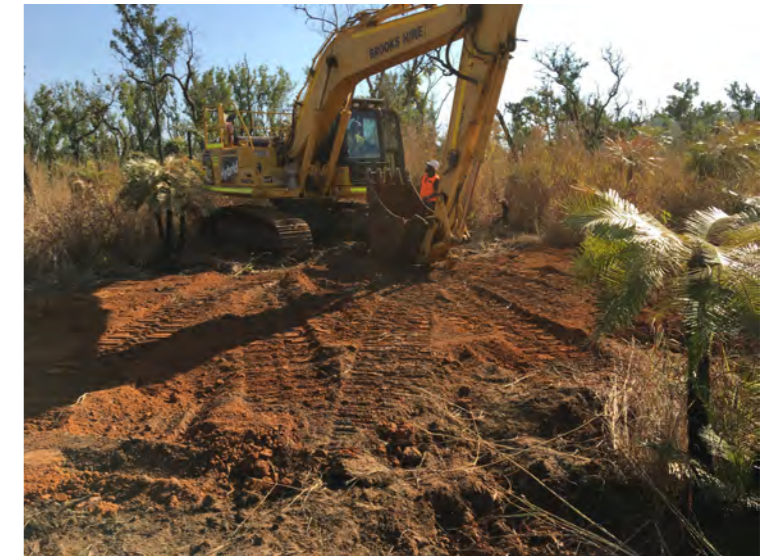
NTP-08 Backfilled Looking South West
