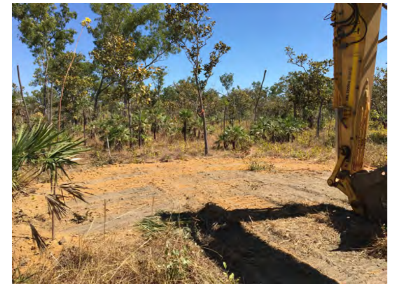
STP-02 Backfilled Looking West
