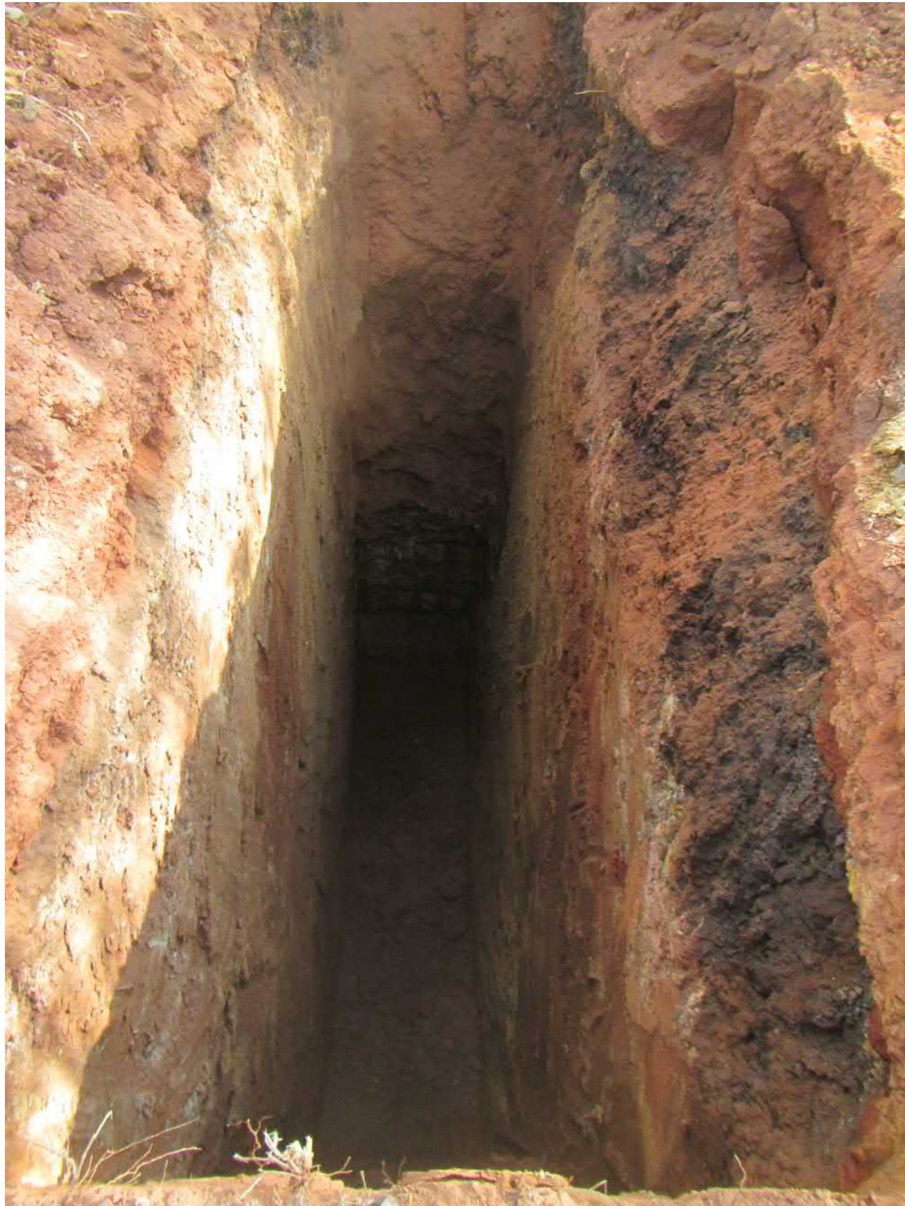
Looking North - Filter Cake in the Eastern Pit Wall
