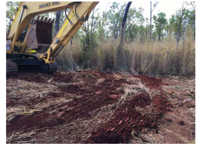
NTP-01 Backfilled Looking South West
