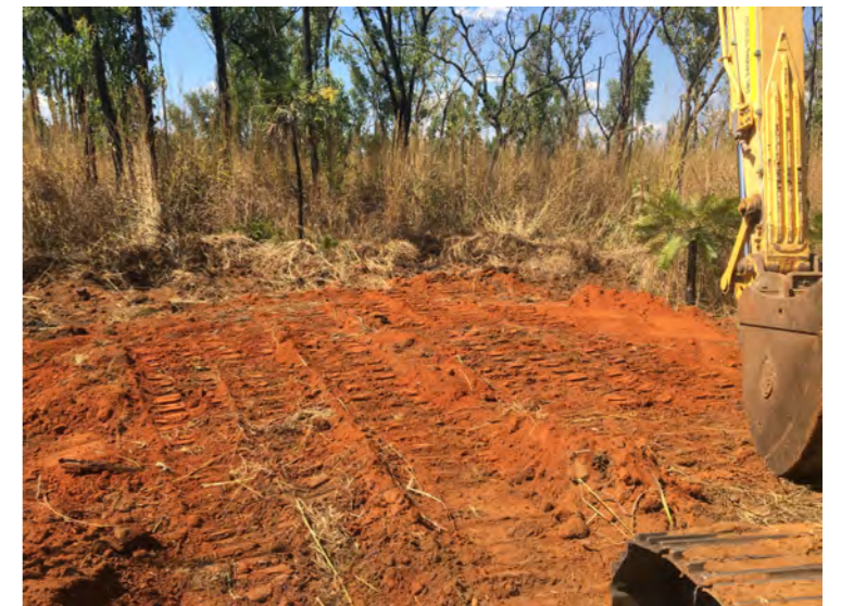
NTP-05 Backfilled Looking North East
