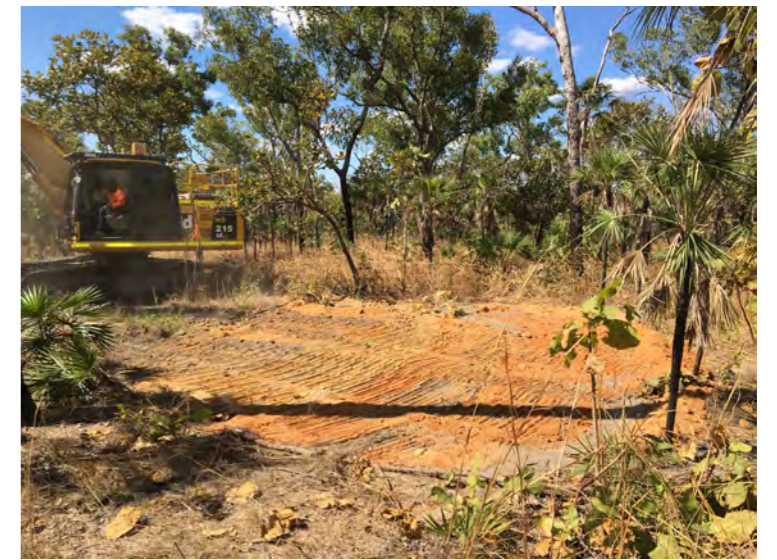
STP-03 Backfilled Looking North East
