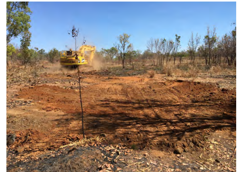
WRTP-14 Backfilled Looking North West
