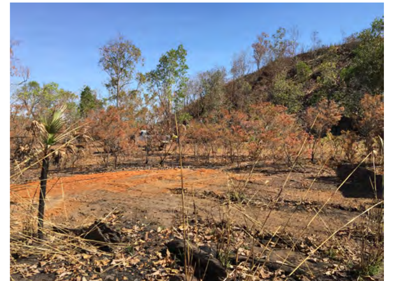
WRTP-20 Backfilled Looking South West
