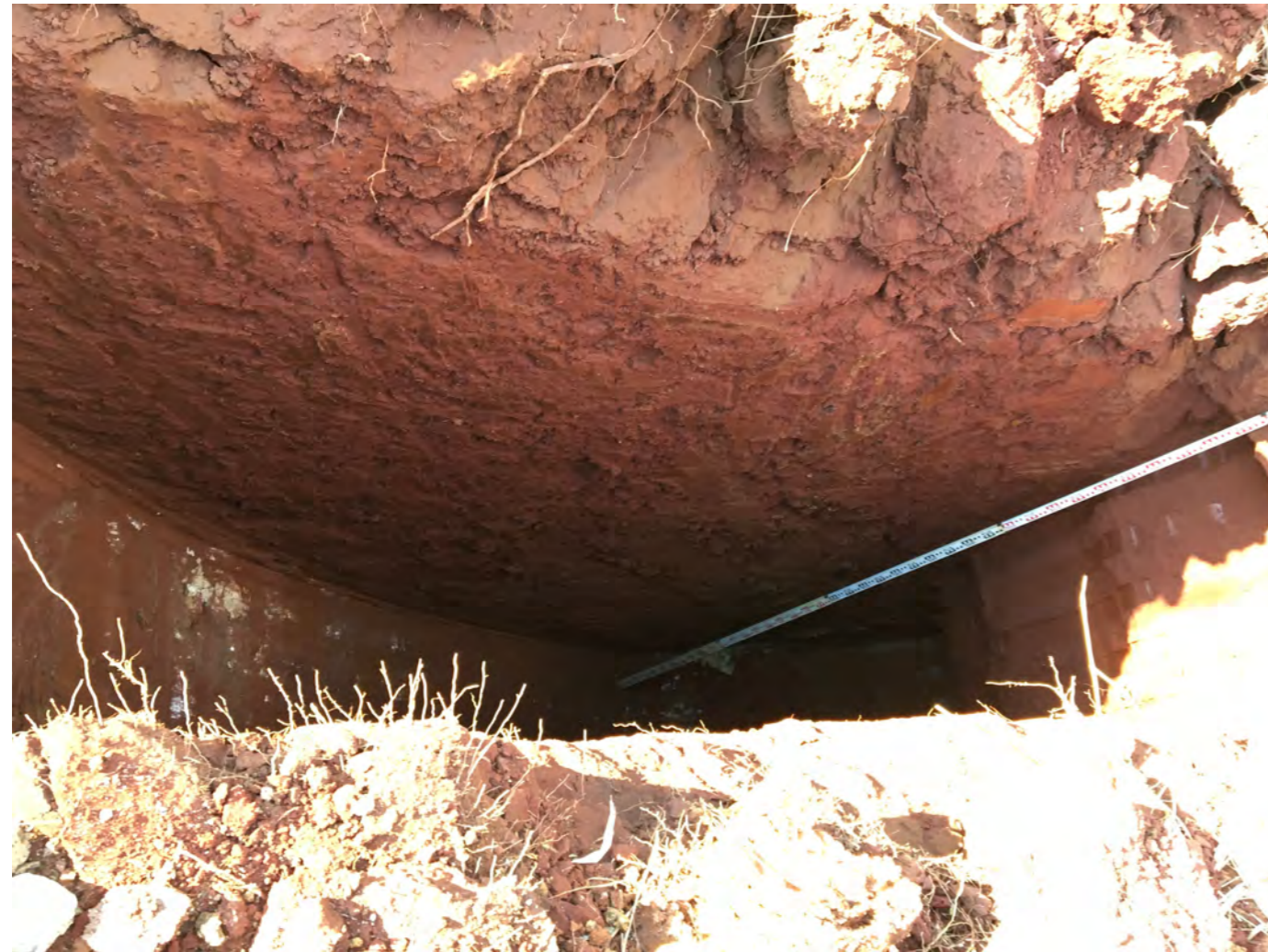
NTP-02 Northern Pit Wall
