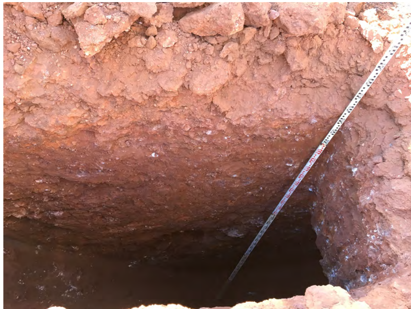
WRTP-17 Northern Pit Wall
