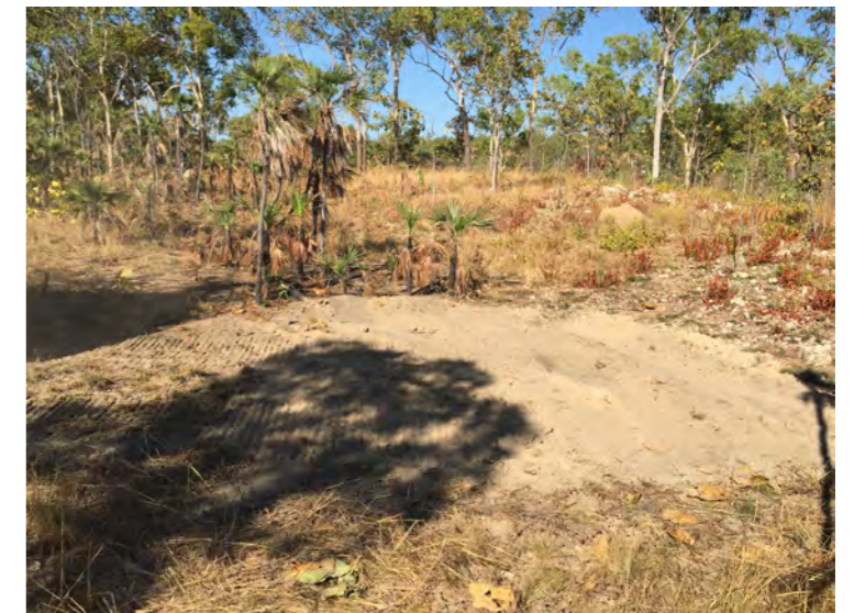
STP-04 Backfilled Looking South West
