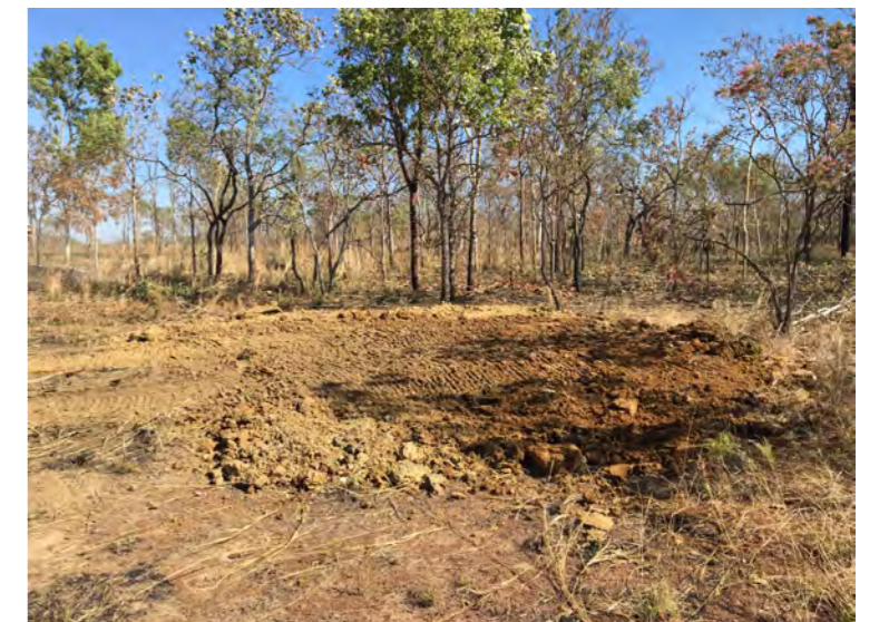
WRTP-16 Backfilled Looking South West
