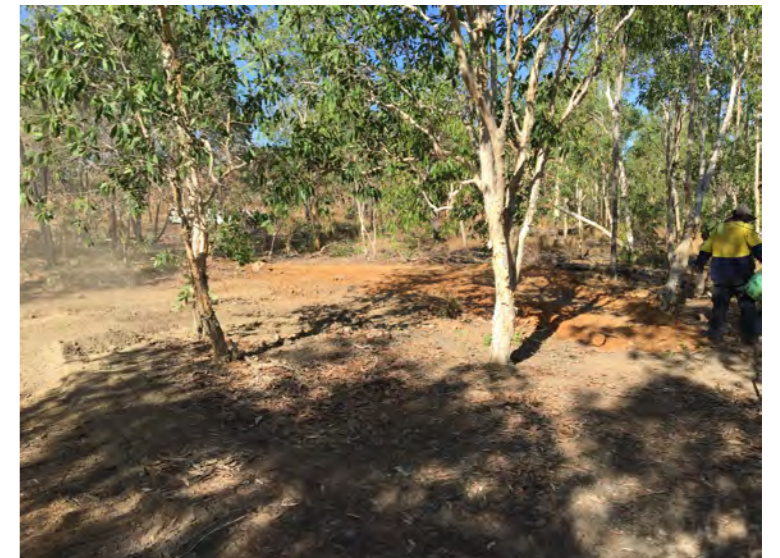
WRTP-19 Backfilled Looking South
