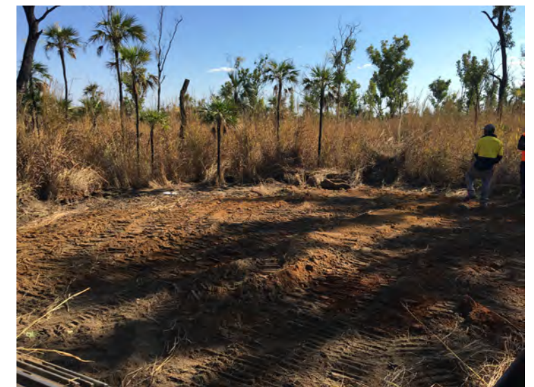
NTP-07 Backfilled Looking North
