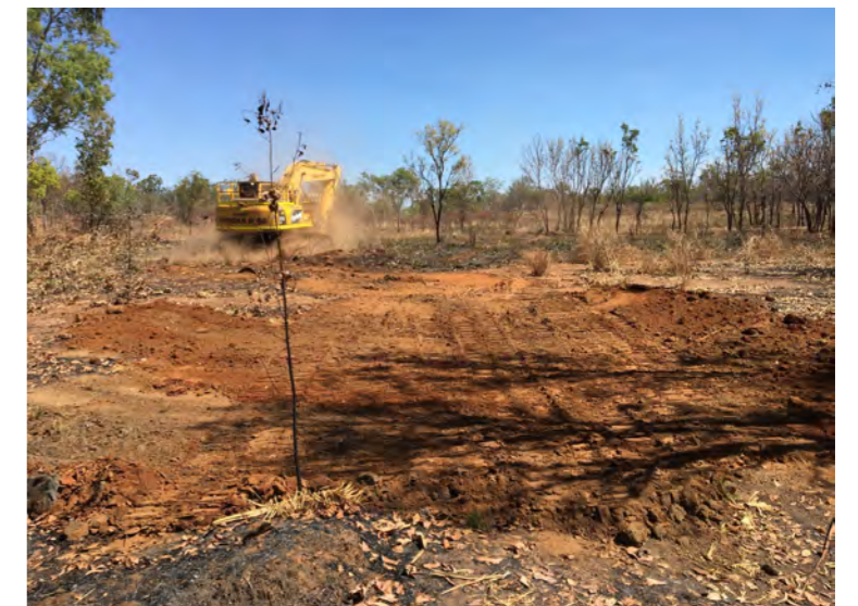
WRTP-15 Backfilled Looking West
