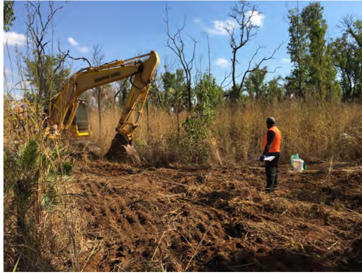
NTP-05 Looking South West
