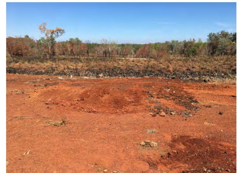
WRTP-18 Backfilled Looking South West
