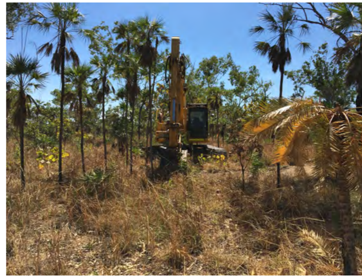
STP-01 Looking North
