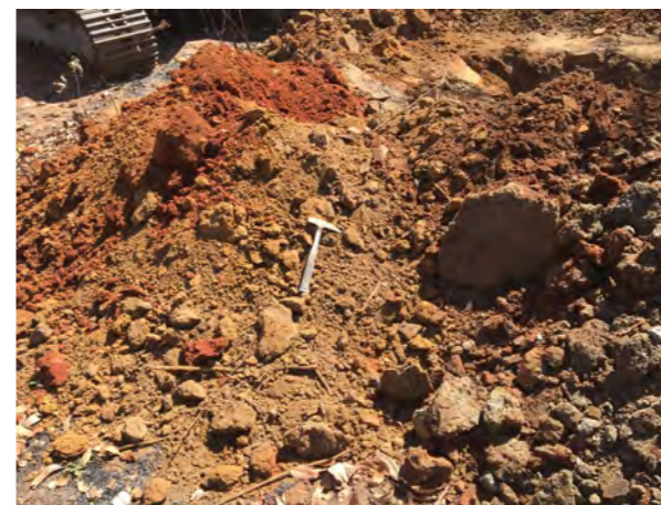
Spoil Pile 0.00m to 1.50m
