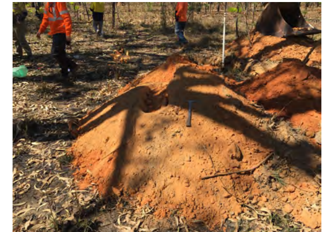
Spoil Pile 0.50m to 1.00m
