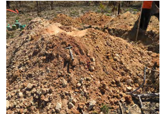
Spoil Pile 2.25m to 3.00m
