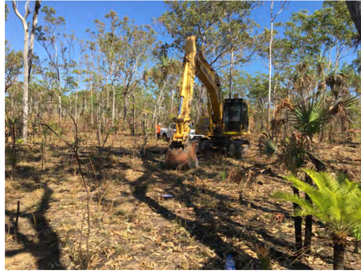
STP-06 Looking South
