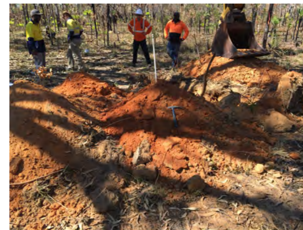
Spoil Pile 1.00m to 1.50m
