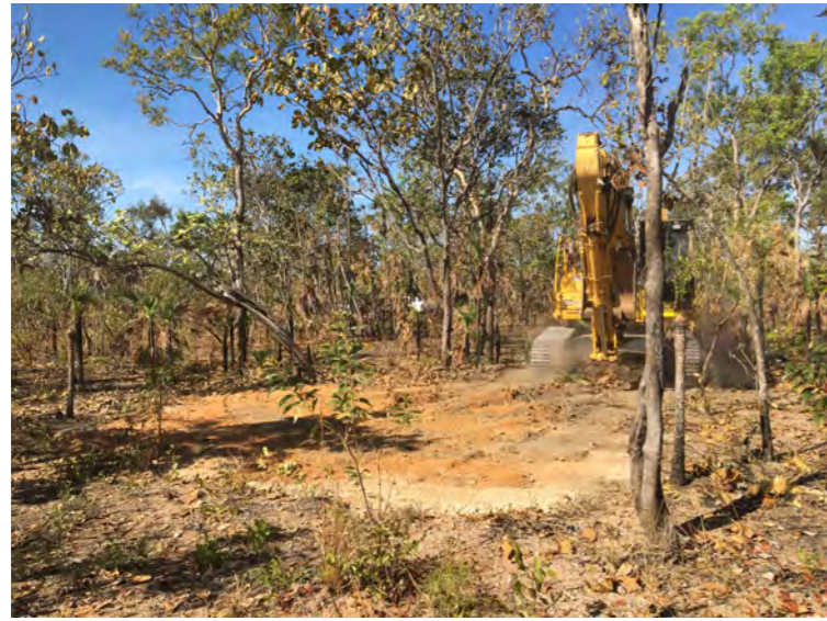
STP-05 Looking South East
