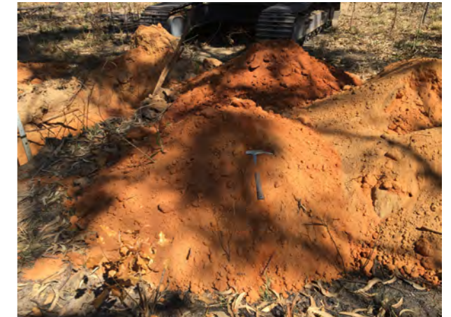
Spoil Pile 1.50m to 2.00m
