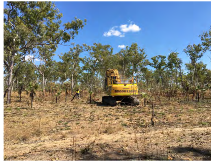
STP-07 Looking West
