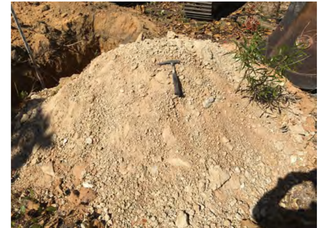
Spoil Pile 1.40m to 2.30m
