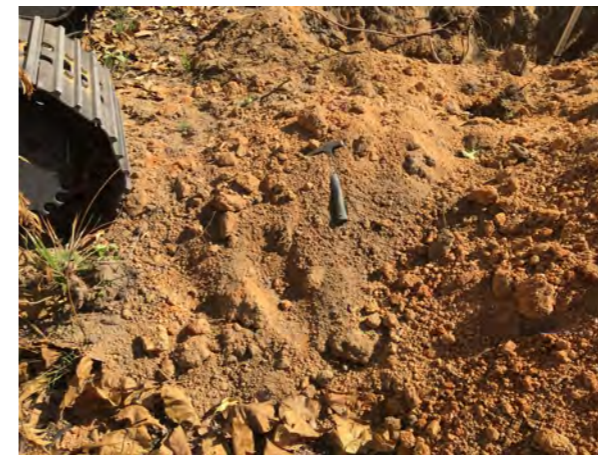
Spoil Pile 0.00m to 0.40m
