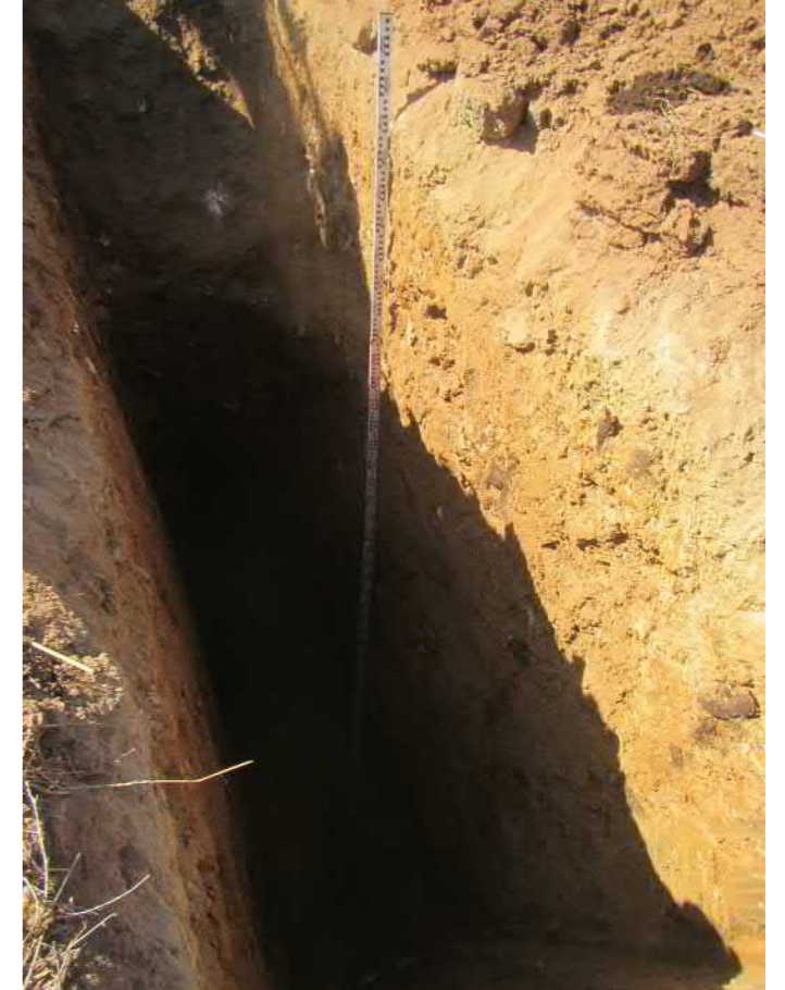
Western Pit Wall
