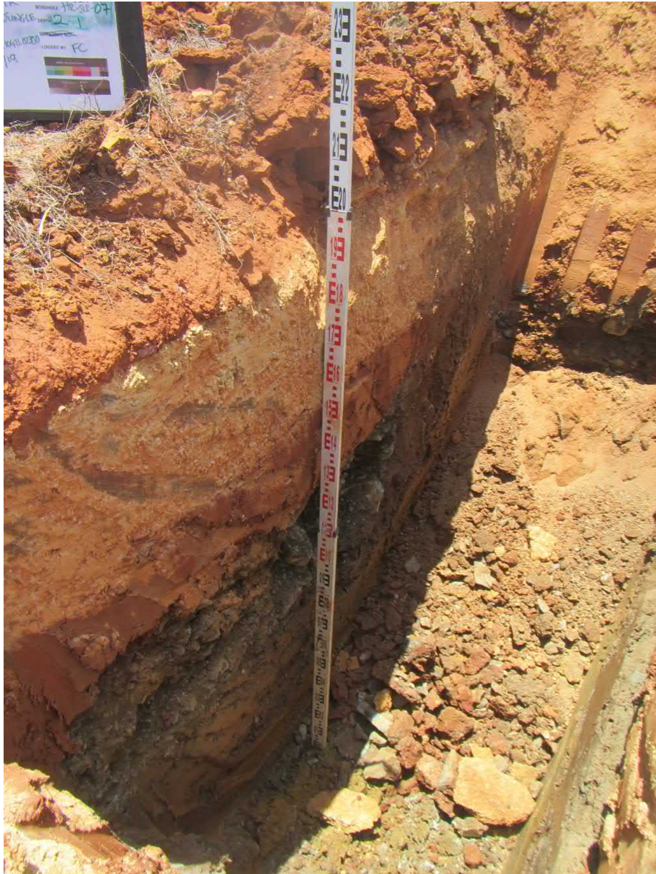
Southern Pit Wall - Gravel Drainage Bed
