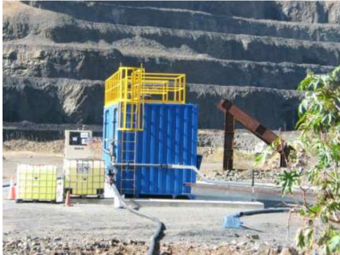
Figure 17 Installation at a quarry
