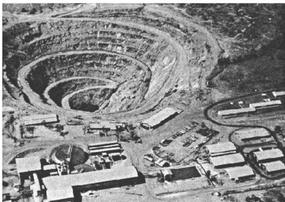
White's Open Cut and Rum Jungle treatment Plant, during the late 1960's. Completed to a depth of 350 feet in 1958.
