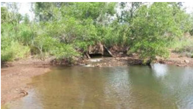
Main Pit outlet April 2015
