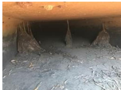
Main Pit outlet August 2019
