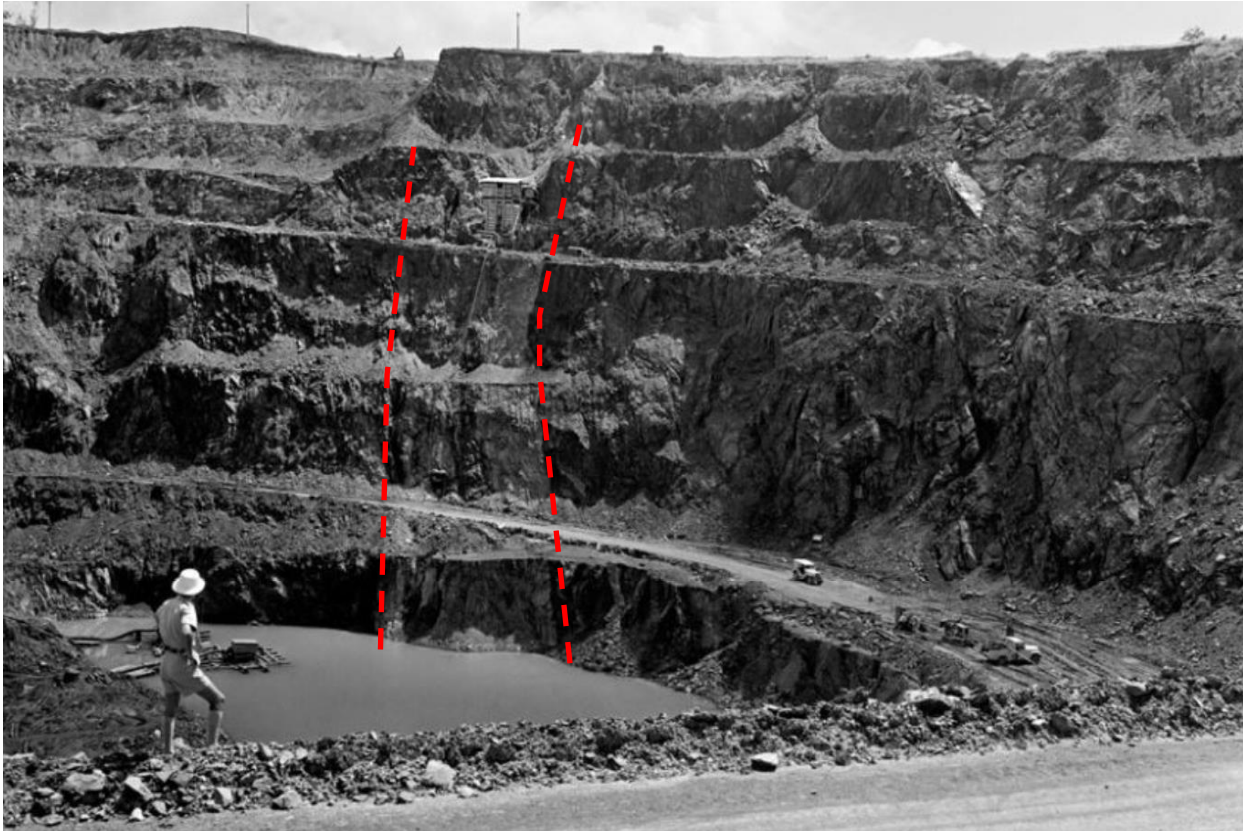
Figure 14 Photograph of White's Open Cut (Main Pit) in 1958 looking north-east along strike of the main shear zone (photo courtesy of National Archives of Australia:A1200,L25494 [8])
