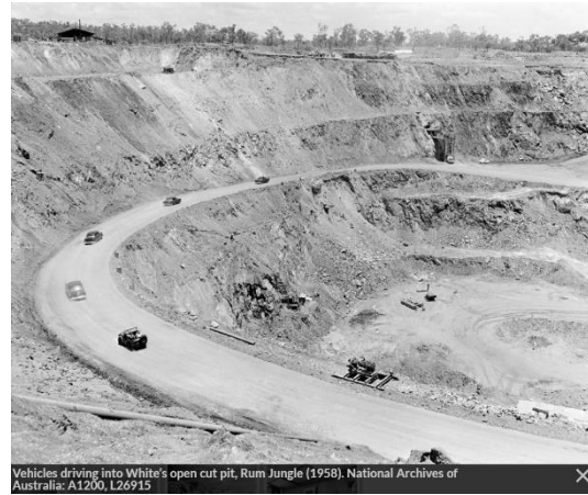
Pit Wall Conditions Looking West (estimated)
