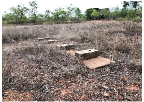
Concrete footings and pads, Rustlers Roost
