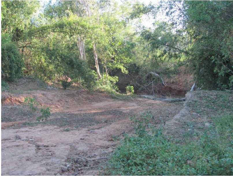
Figure 4-1 Cattle crossing installed at MBC01.
