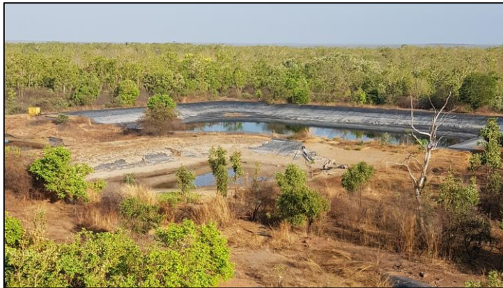
Plate 1-7 Remaining Heap Leach Pond at Quest 29
