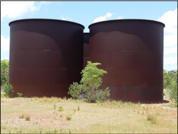
Plate 1-2 Remaining Tanks from Former Processing Plant at Rustlers Roost
