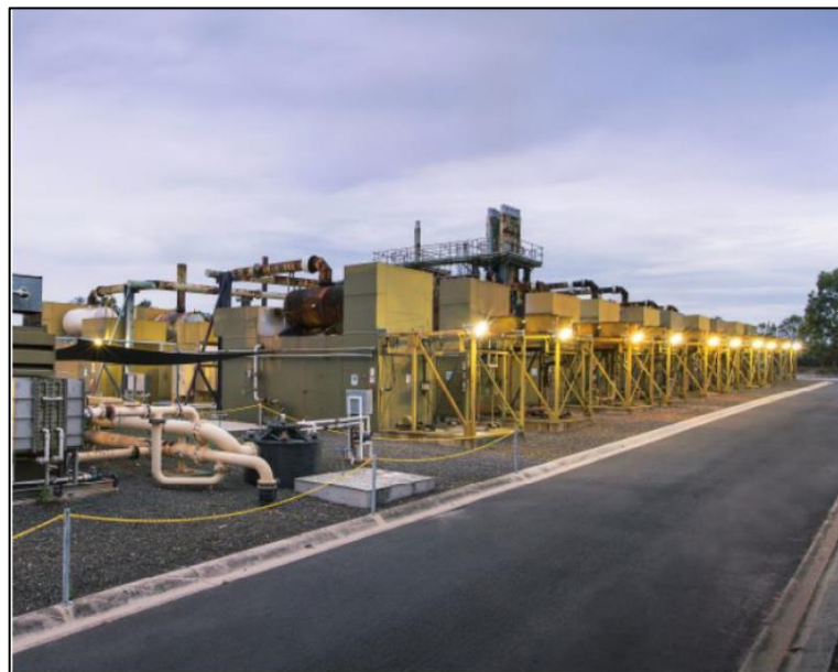
Plate 4-1 Indicative Power Station
