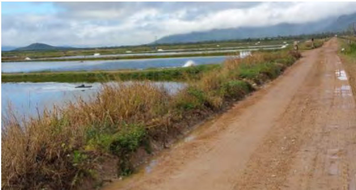
PLATE 9 TRAFFICABLE BERMS IN EXISTING SEAFARMS' OPERATIONS
