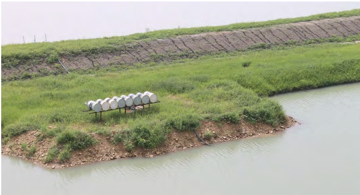
PLATE 8 EMBANKMENT PROTECTION AGAINST EROSION, JANUARY 2017
