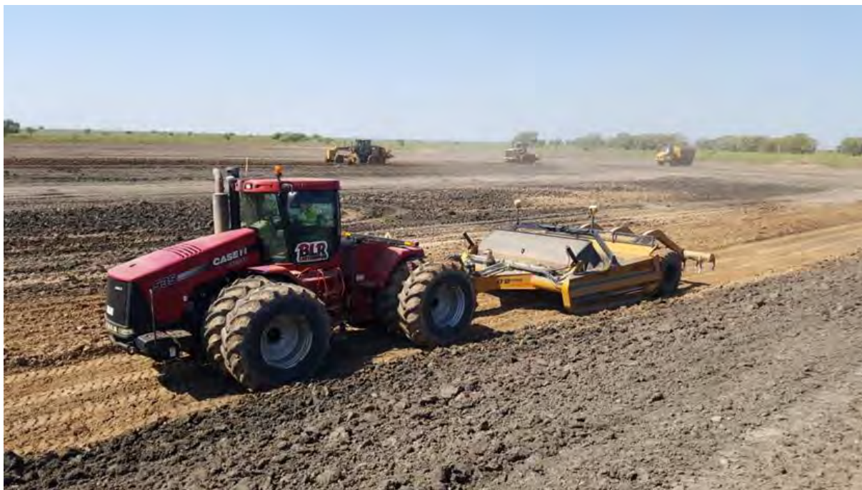
PLATE 1 EARTHWORKS TRIAL IN PROGRESS
