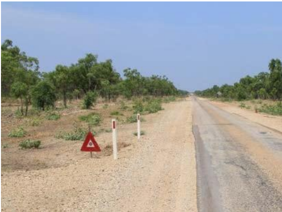
Figure 2 – Culvert headwall within 2.5m of edge of seal
