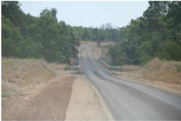
021 20km Salt Ck Bridge Outbound.JPG
