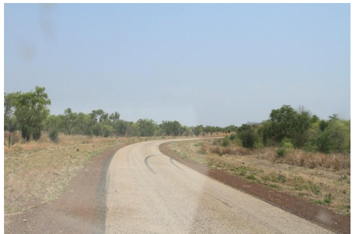
Figure 3 - Curve at Approx. Ch58
