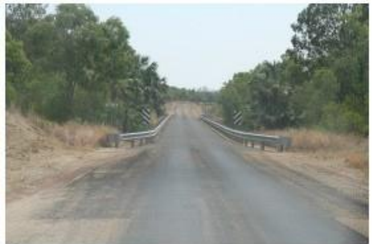
025 20km Salt Ck Bridge Outbound.JPG
