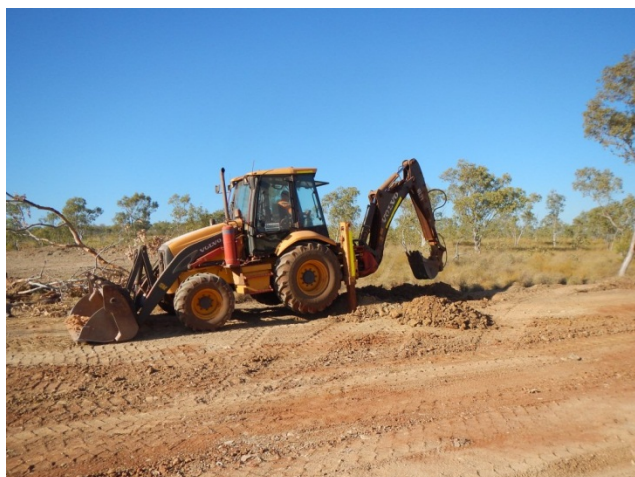
Figure 3-2. Photograph of soil pit excavation
