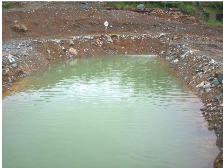
Figure 3-3: Example of a Sediment Basin (photo: http://krominco.com/ )
