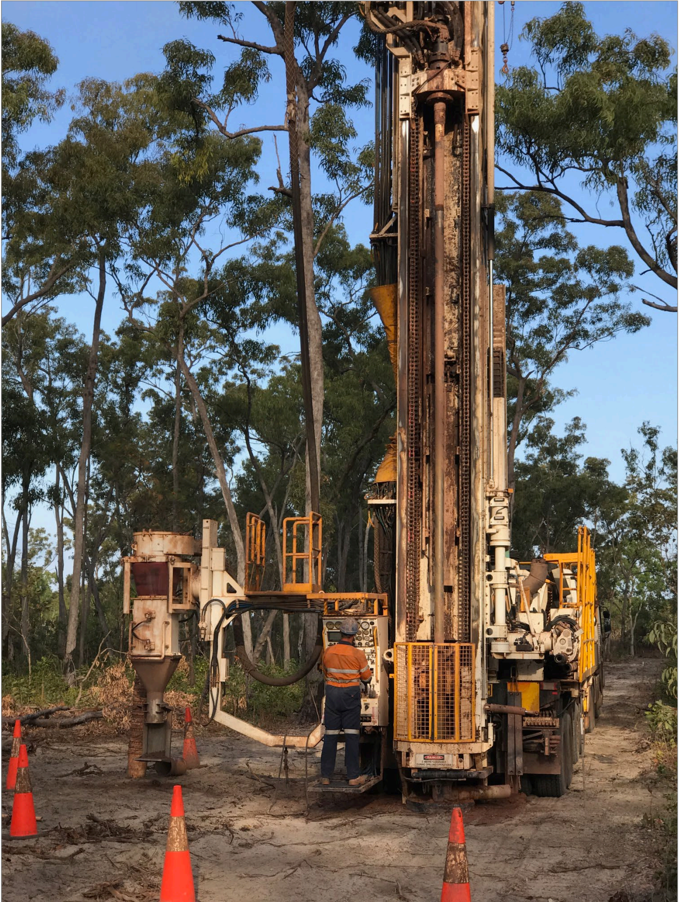
Photo 2-1 Example of a Reverse Circulation Drill Rig
