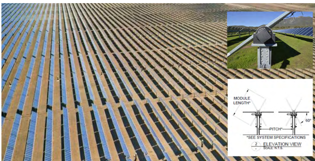
Figure 2-4. Photograph of single axis solar tracker arrays
