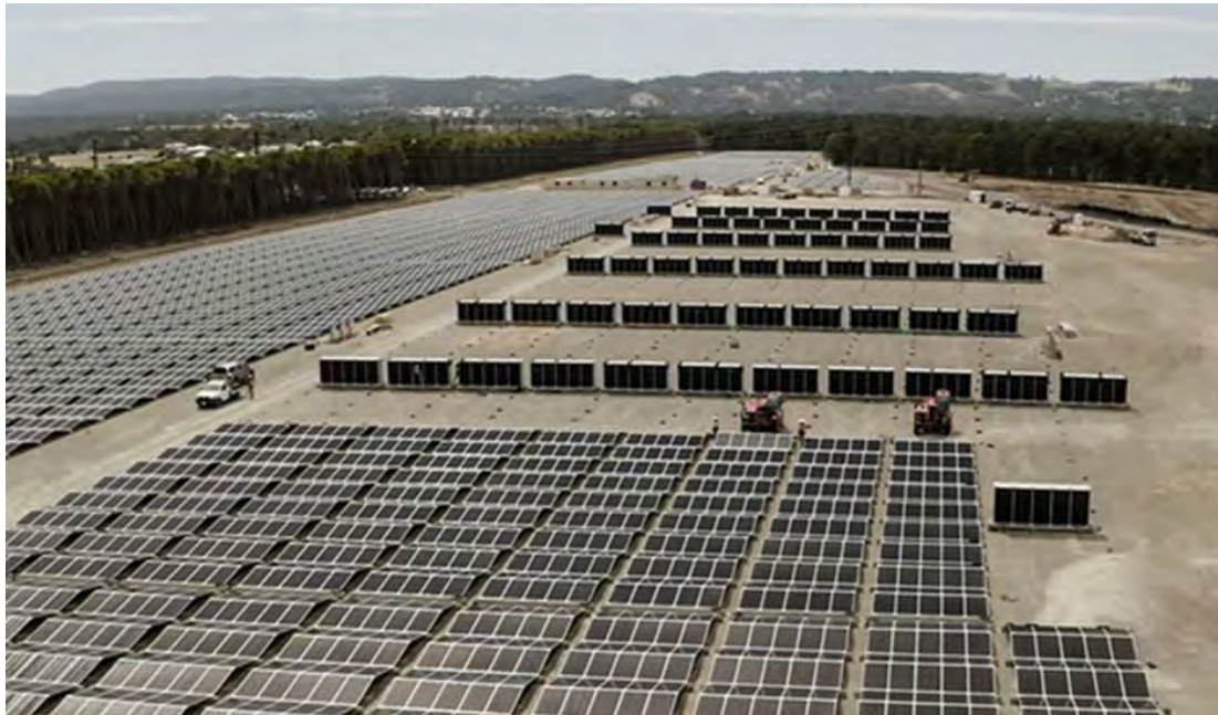
Figure 2-3. Photograph of fixed tilt solar panel arrays
