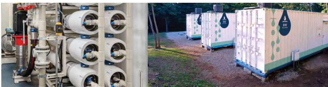
Figure 5-2. Photograph of a temporary containerised desalination facility
