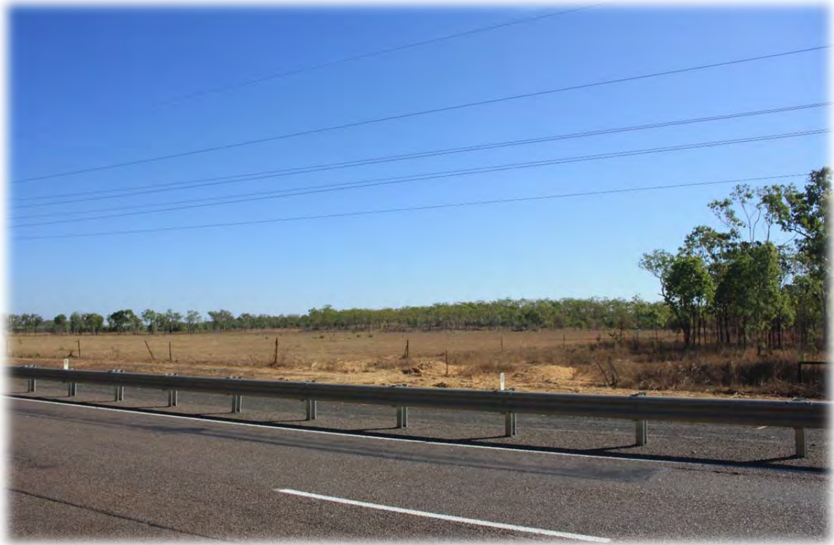
Figure 54: Arnhem Highway - Southern side of Mount Bunday Creek looking southwest towards the TGU Project
