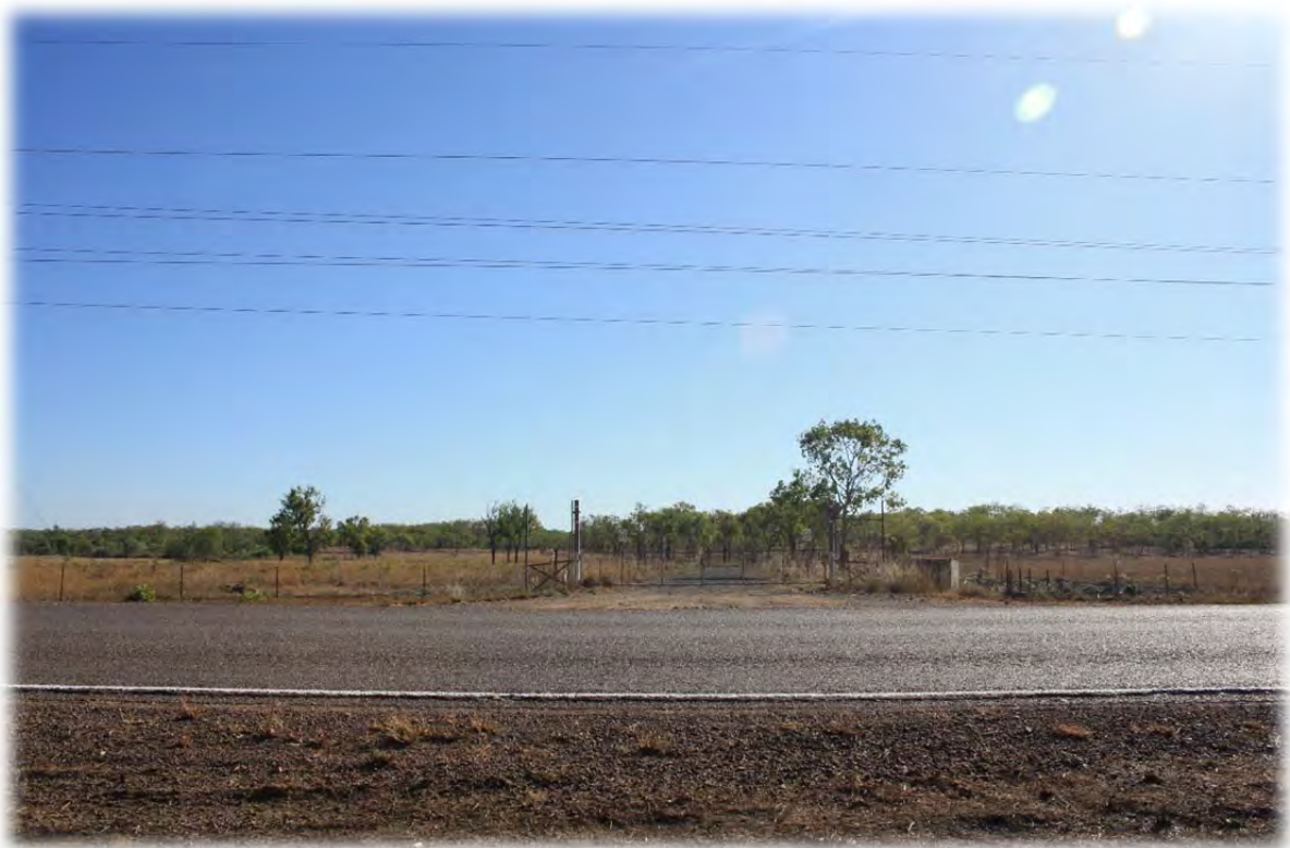
Figure 55: Arnhem Highway – Looking west along the TGU Project access road
