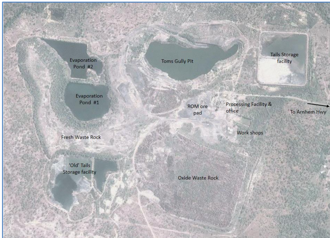
Figure 2: Toms Gully Mining Infrastructure
