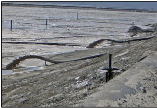
Photo 1: Photograph showing typical spigot arrangement and tailings discharge.
