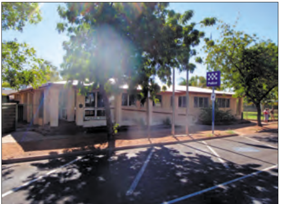
Plate 6.3 Tennant Creek police station
