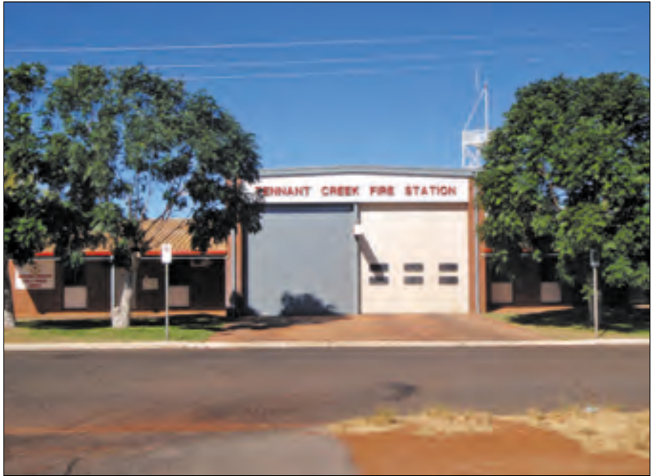
Plate 6.4 Tennant Creek fire station
