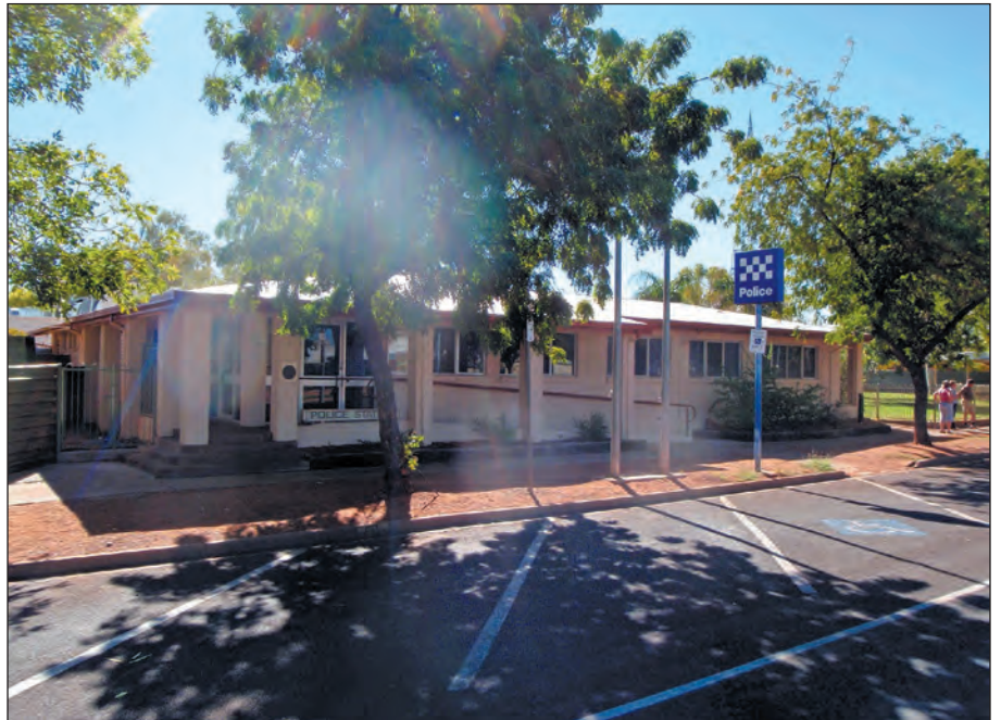
Plate 5.6 Tennant Creek police station
