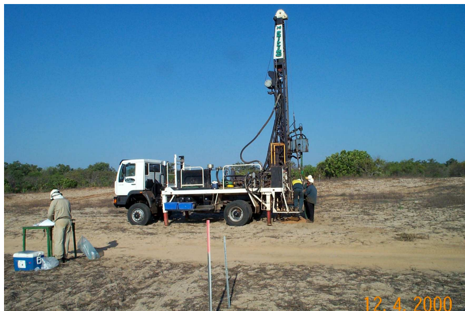
Plate 6: Drilling of OSA17 (Geotechnical Bore ID: P/BH6) near the tree-line.
