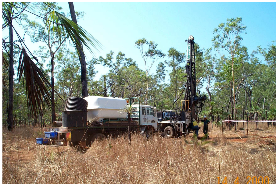
Plate 15: Drilling of OSB25 (Geotechnical Bore ID: G/BH2) within the proposed plant site (Area B).
