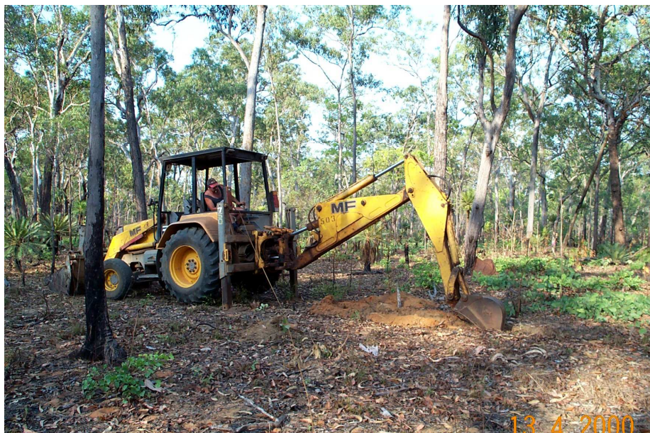
Plate 11: Backhoe digging test pit location OSB20 (Geotechnical Bore ID: P/TP12) within Area B.
