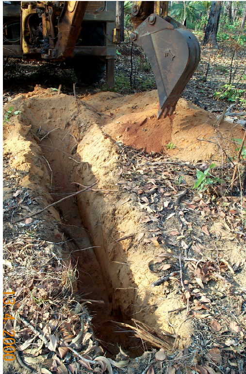
Plate 12: Completed test pit OSB20 (Geotechnical Bore ID: P/TP12) along the proposed pipeline corridor of Area B.
