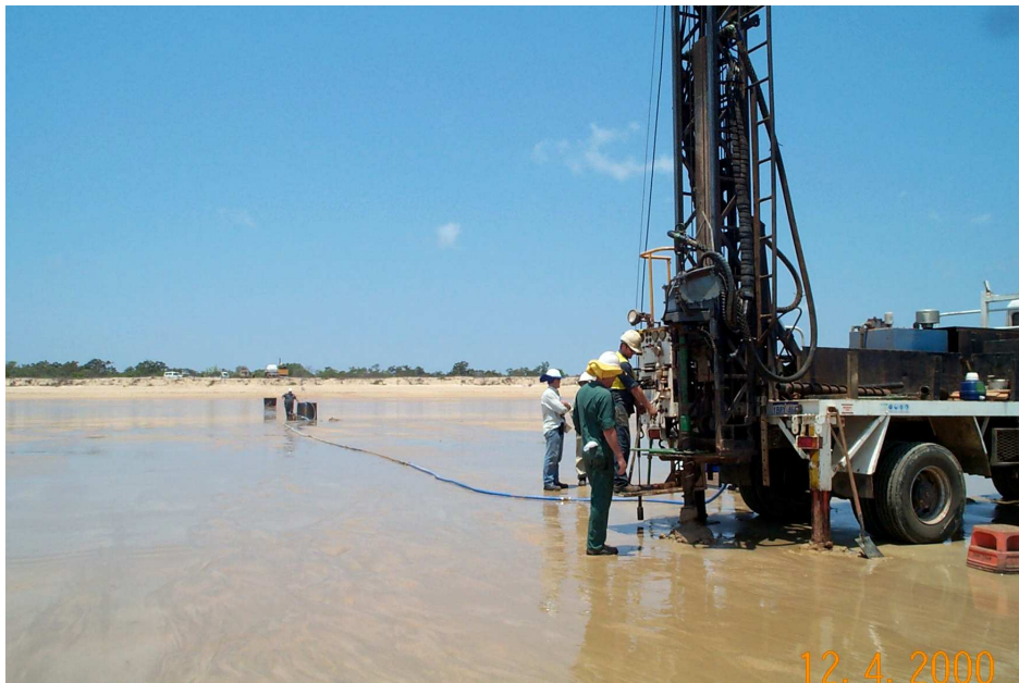
Plate 1: Drilling at location OSA12 (Geotechnical Bore ID: P/BH4).
