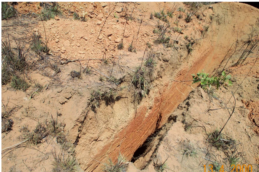
Plate 9: View into test pit location OSB18 (Geotechnical Bore ID: P/TP14) along the proposed pipeline corridor of Area B.
