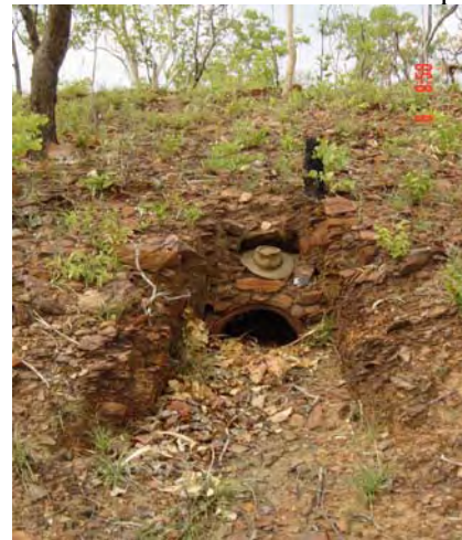
Drain, facing west
