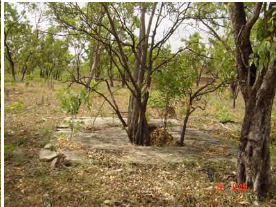
One of the concrete floor slabs on lower slope
