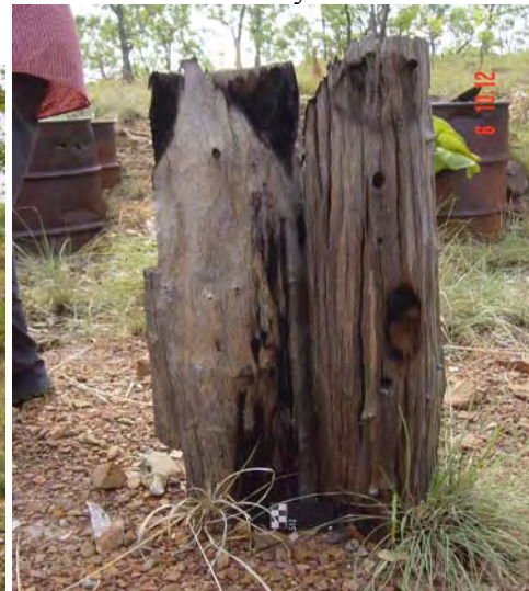
Close up of a timber pole
