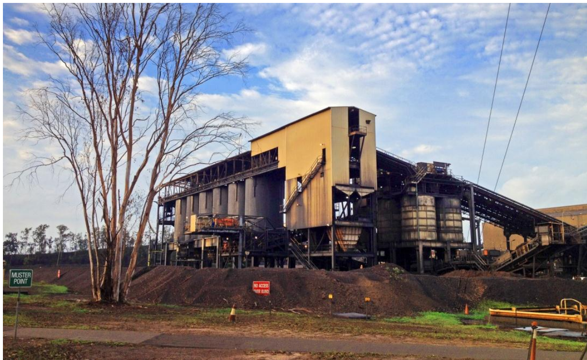
Plate 4 View of Concentrator at the Existing GEMCO Mine
