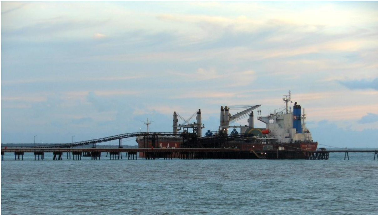
Plate 5 View of Wharf at Milner Bay Port Facility
