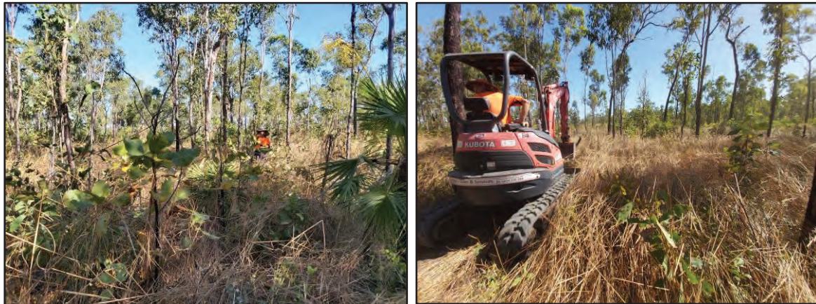
Figure 3-6 Overview of surrounding of locations TP07 during location mark up and underground service clearance.
