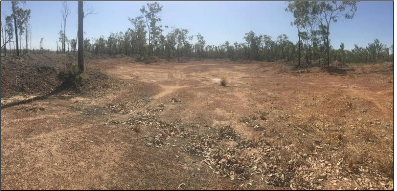
Photograph 3: Excavation/soil stockpile area in northern portion of Site (panoramic)
